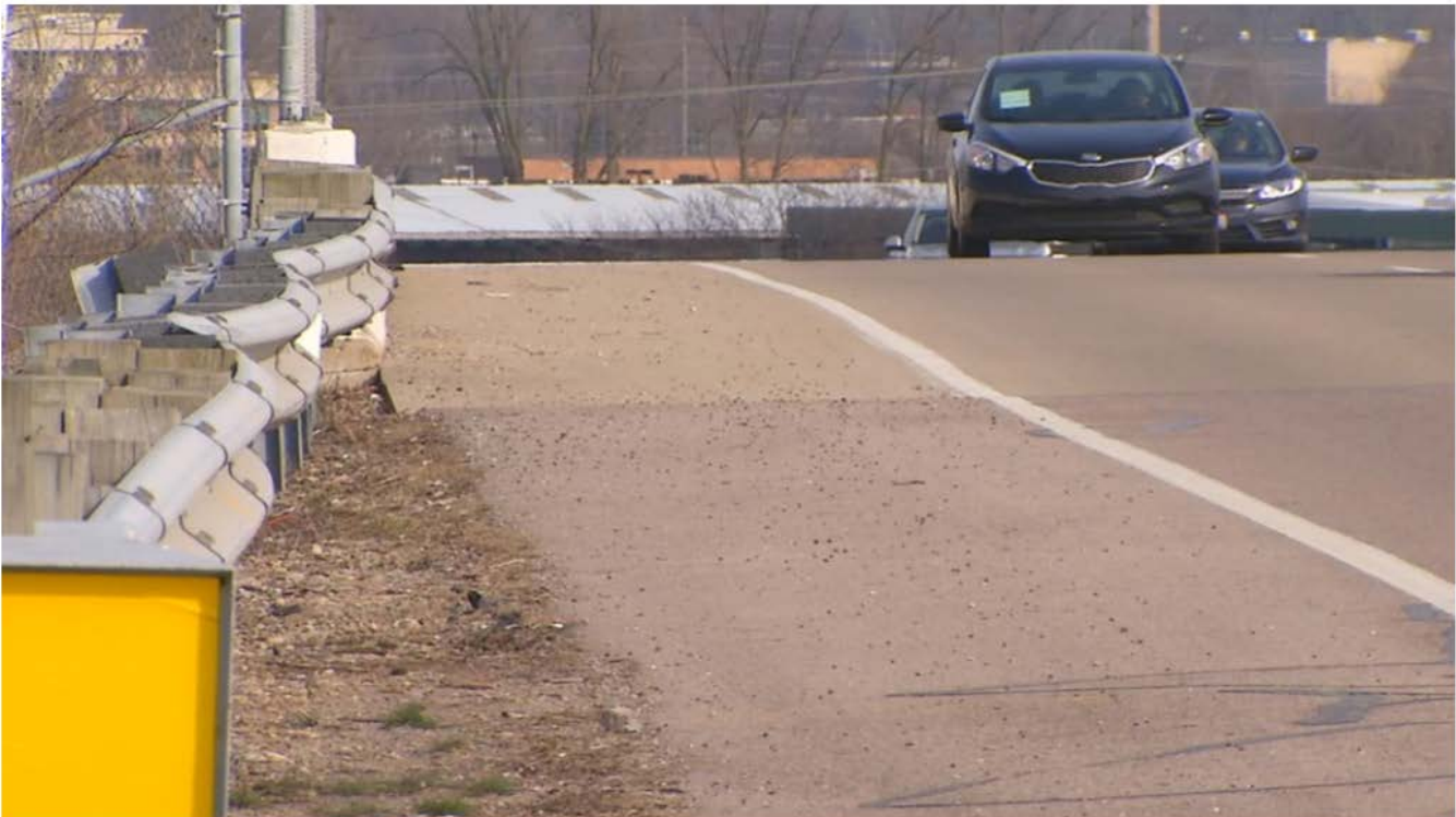
Work to begin on pedestrian access project near Dayton Mall (File: WKEF/WRGT)
